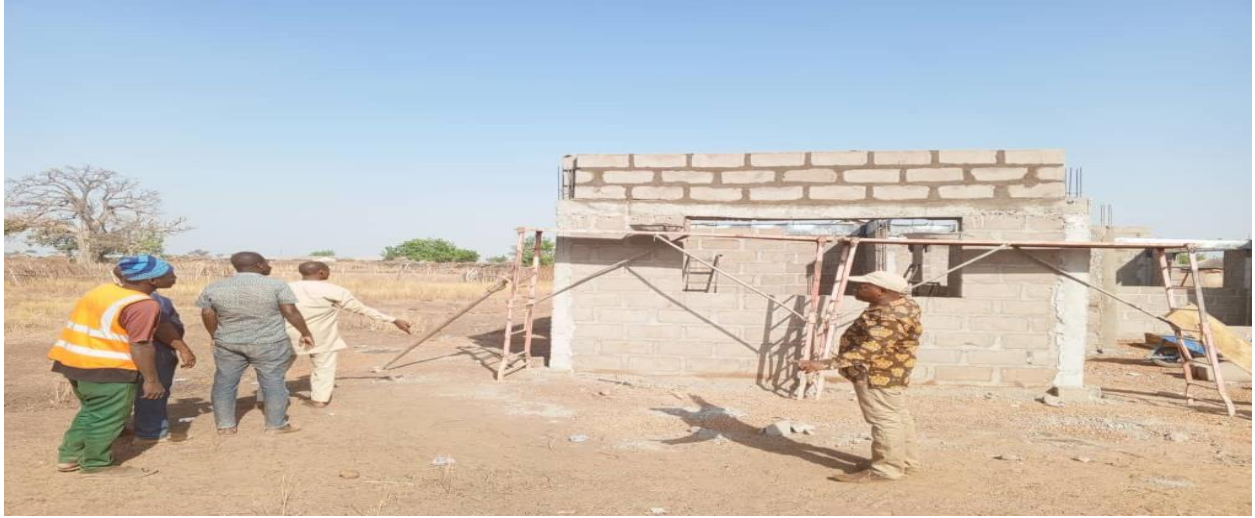
MATERNITY BLOCK AT BAGLI CHPS FUNDED BY MP'S NHIL
