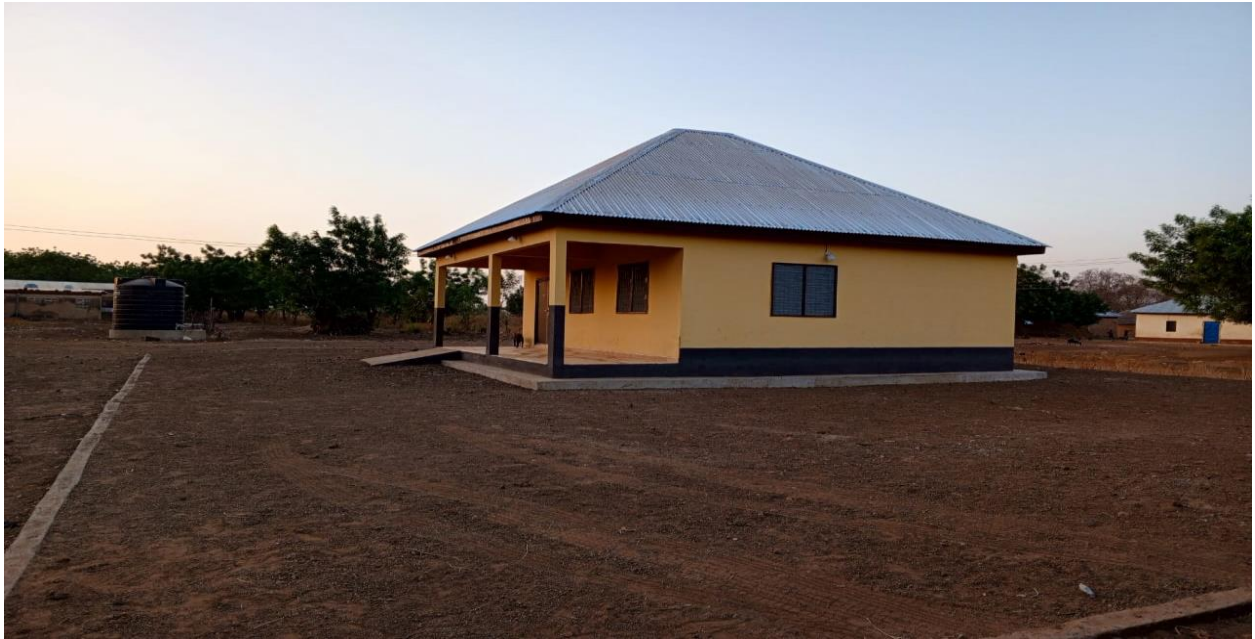
ICT CENTER AT PISHIGU UNDER SOCO
