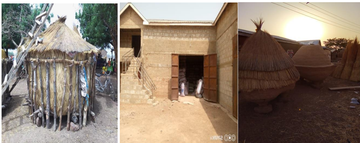
Samples of thatched Silo (left), warehouse (middle) and clay 'Buli' for storage of farm produce
